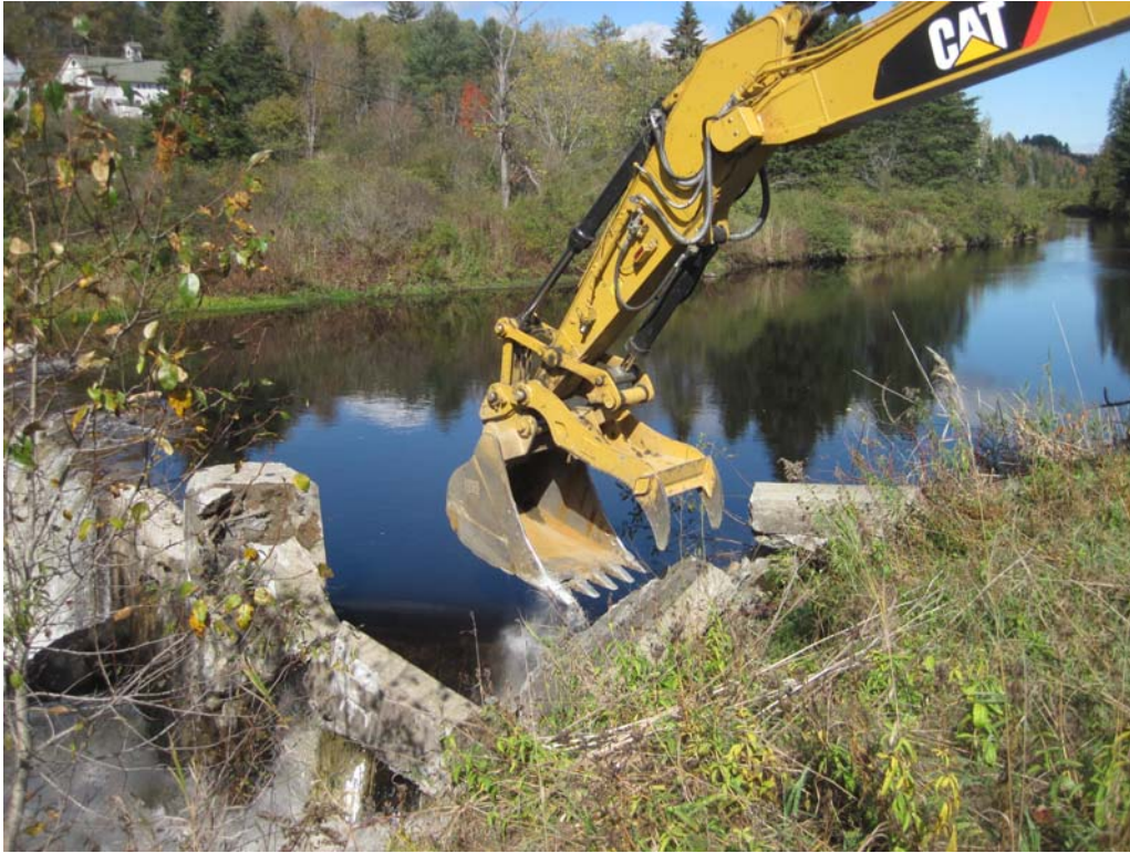
Removal of the top of the former sluice gate.
