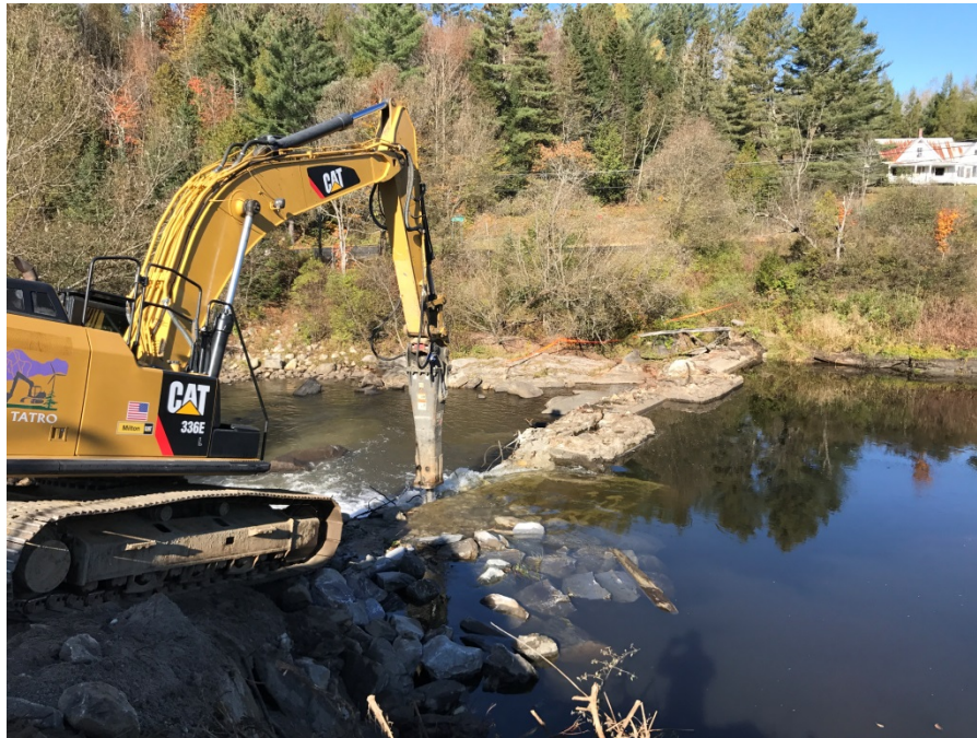
Continued dam removal and lowering water level.
