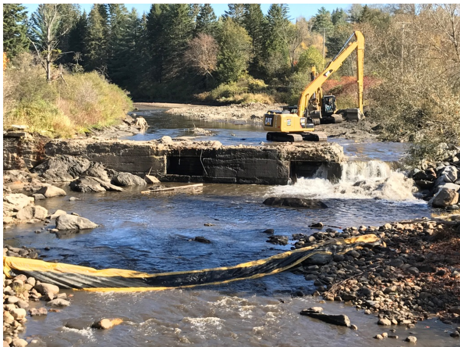
Dewatering and Sediment removal.
