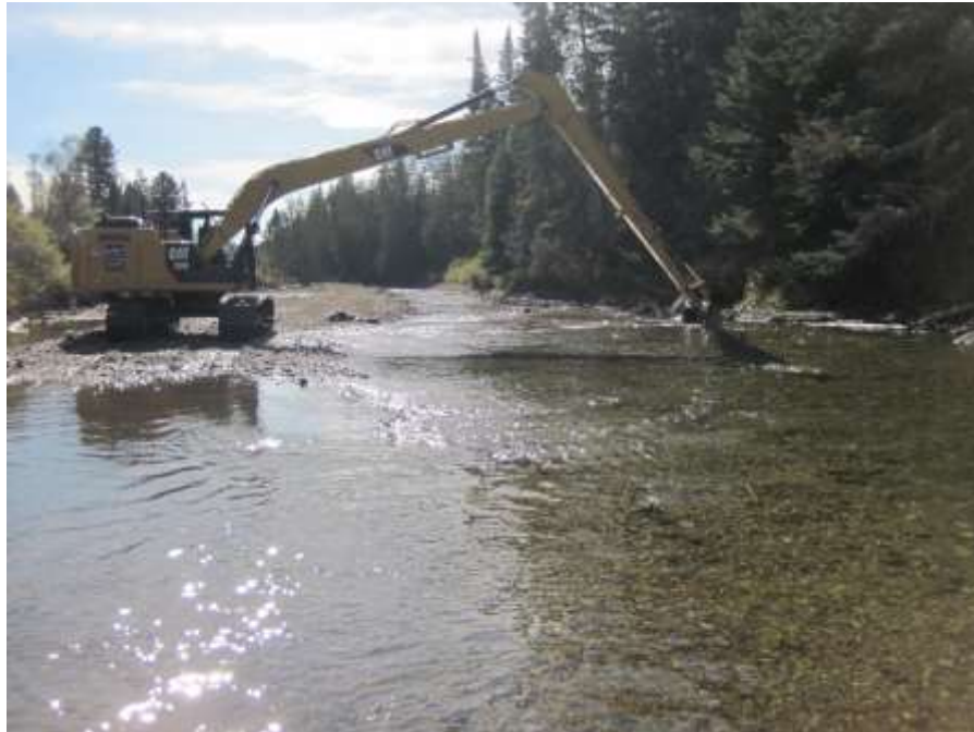
Sediment removal at upstream extend of project.
