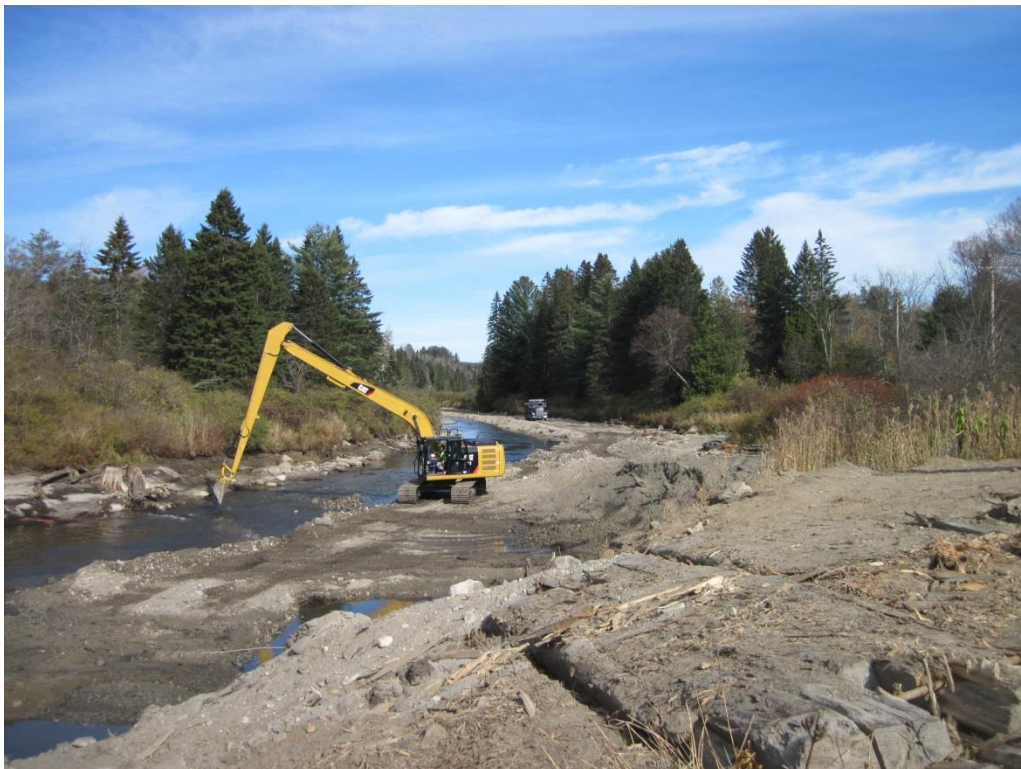
Sediment removal and hauling on stockpiled material removed from channel.
