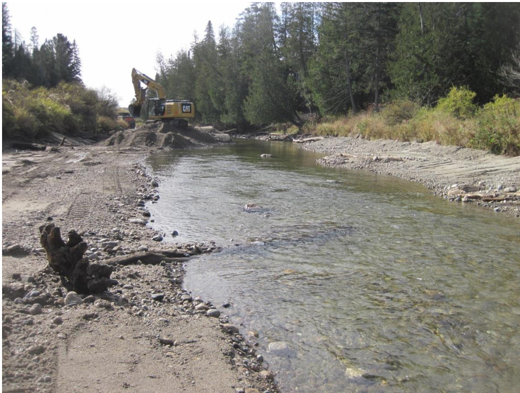
Restored channel and flood benches near upstream end of project.
