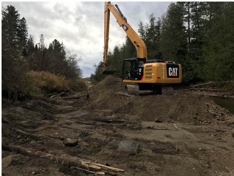
Sediment removal from floodplain.
