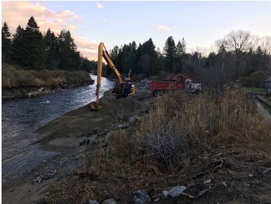
Loading and hauling sediment removed from in front of dam after high water.
