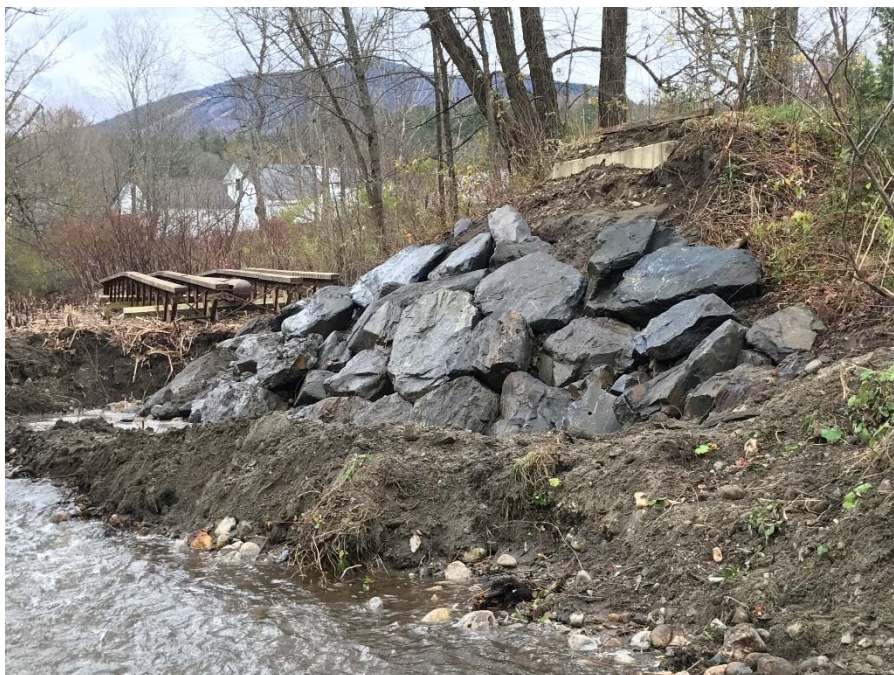
Armored river left (facing downstream) bridge abutment with bridge removed.
