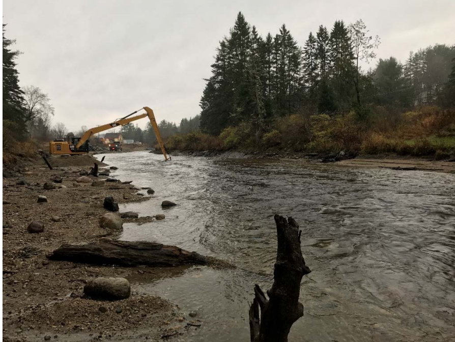
Continued sediment removal and channel/floodplain restoration.
