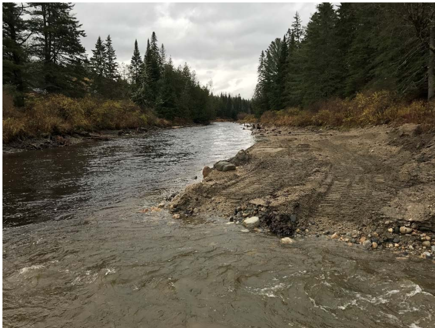
Partially restored channel under high flow.
