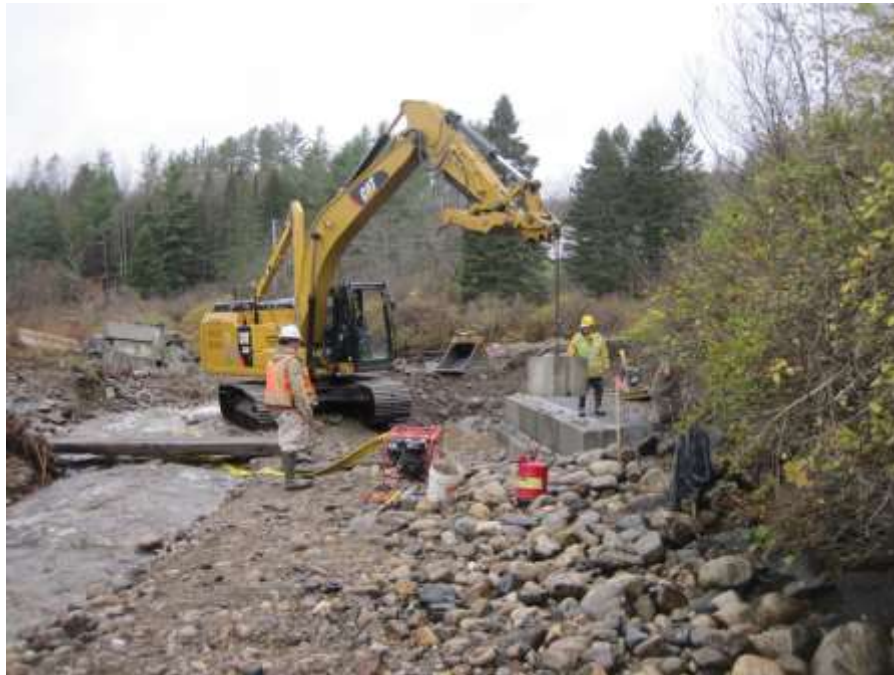
Installed right abutment on Dish Mill Brook (looking downstream).
