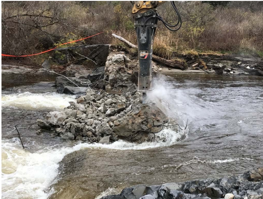
Concrete removal.
