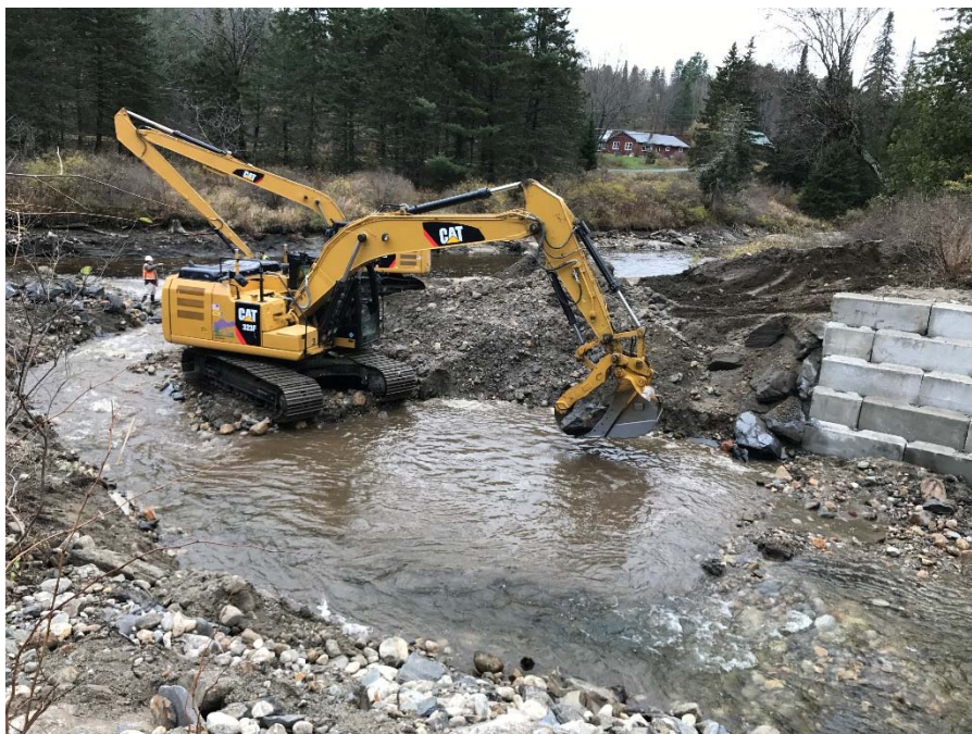
Bed armor installation on Dish Mill Brook.
