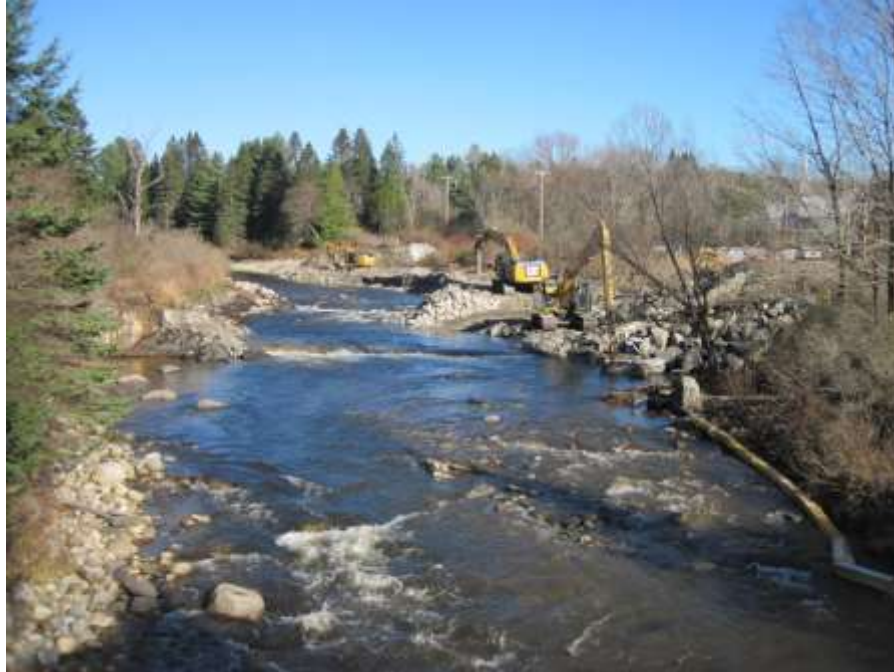
Concrete removed down to low apron.
